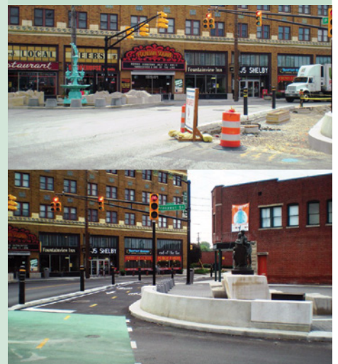
Fountain Square construction near completion in September 2012.
