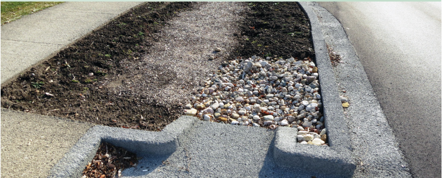
Central Greens green infrastructure near completion.
